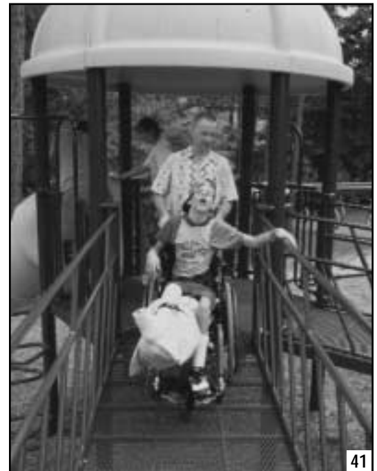
The 80-inch vertical clearance height does not apply to elevated accessible routes. This allows for the use of features such as roofs and sun shelters.
