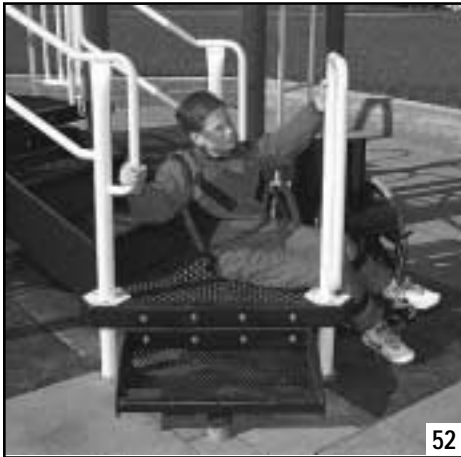
Materials in a variety of different shapes and sizes are used to manufacture transfer supports including metal, plastic, and rope.
