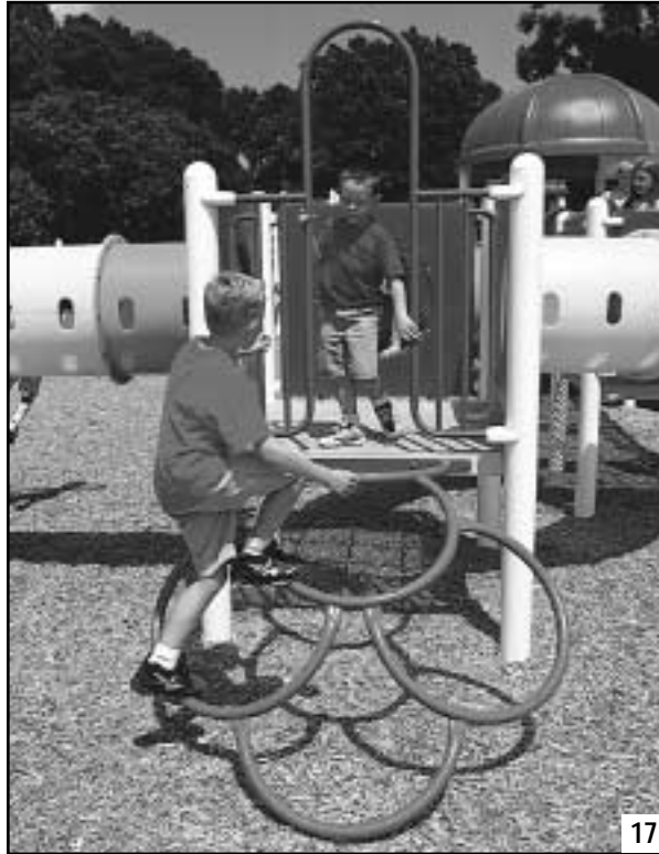
This climber is considered an elevated component, since it can be approached or exited from the ground level or above grade from a platform or deck on a composite play structure.
